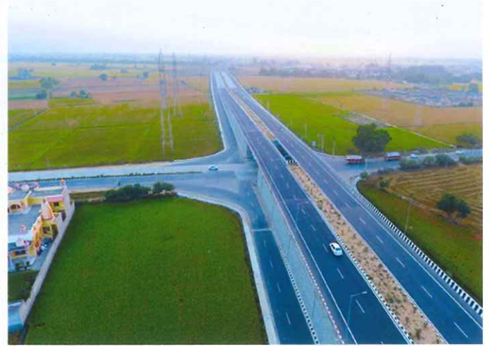
Sangrur Bypass Project, Punjab
