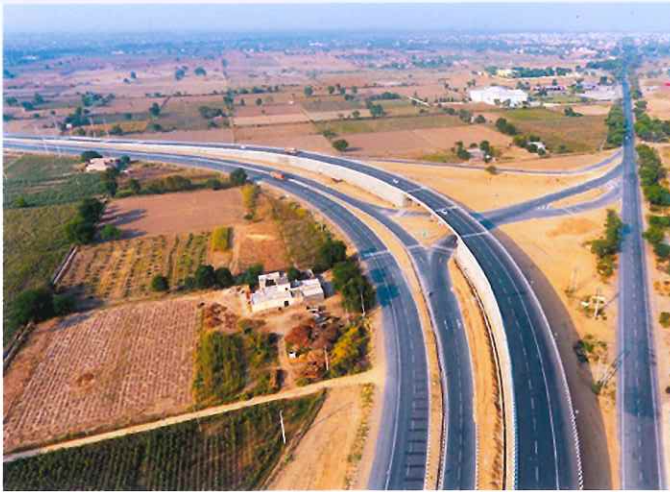
Kaithal road project, Rajasthan
