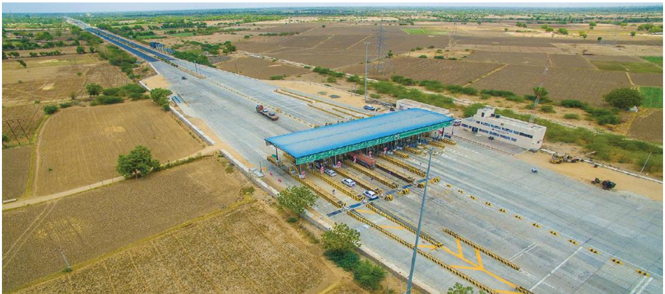
Bhalgam Toll Plaza
