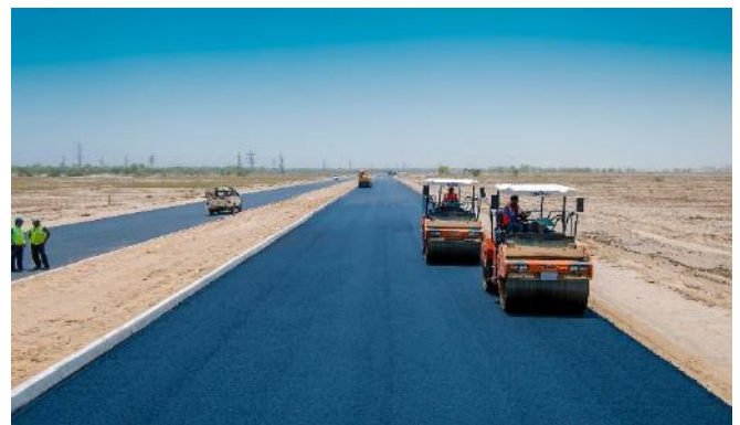
Bituminous Layer Compaction on Kaithal-RJ Border Road Project
